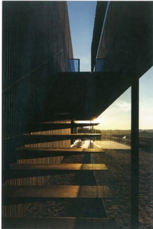
Casa Principal Main House Escadas exteriores Stairs details
